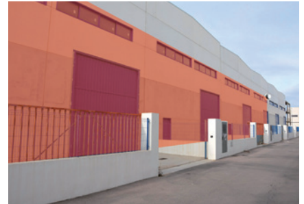
Wall protection (outdoor) at Warehouse
